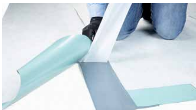
Sealing by butyl tape RENOLIT ALKORPRO BAND
