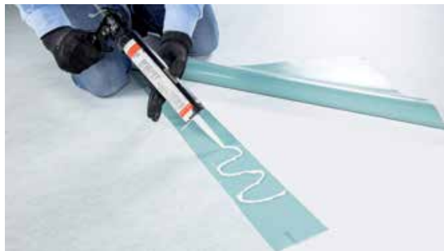
Sealing by mastic glue RENOLIT CEM 805
