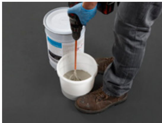
4. Mix thoroughly (2 to 5 min., depending on the temperature).
