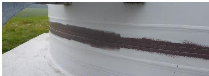
Primer applied to both welded seams
