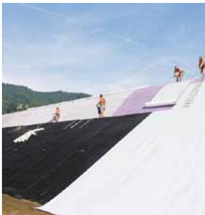
Waterproofing system-intermediate fixation
