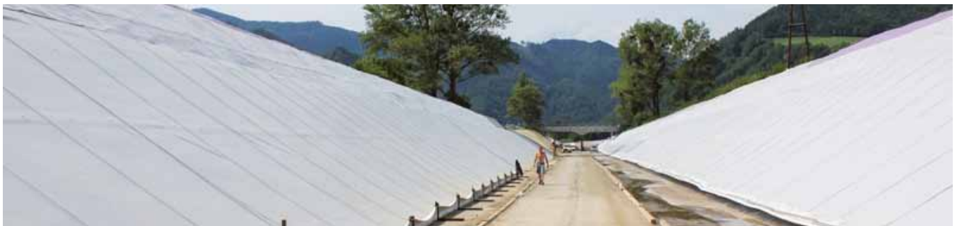
Unrolling and placing of geomembrane
