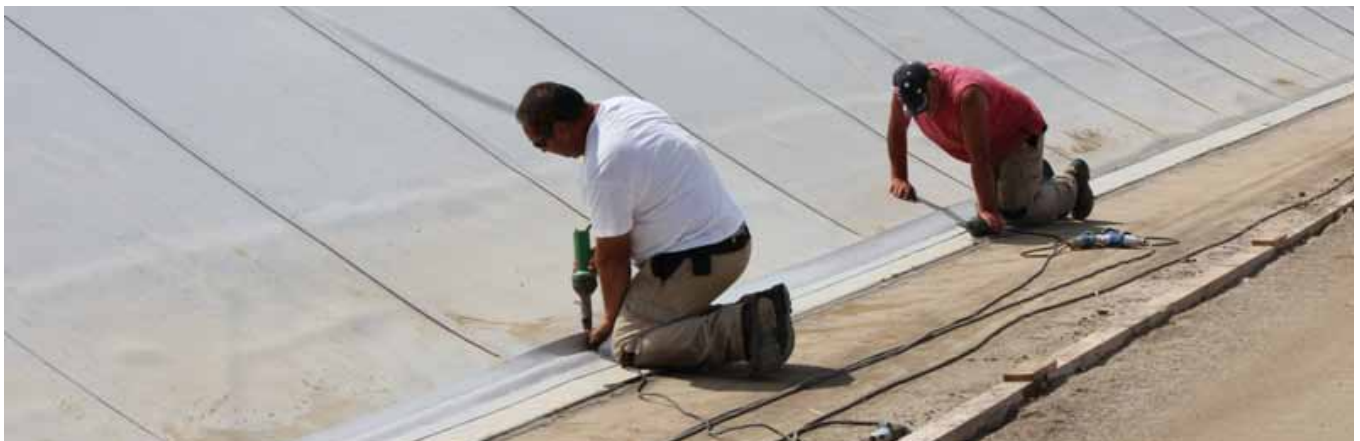
Welding with hot air and double seam
