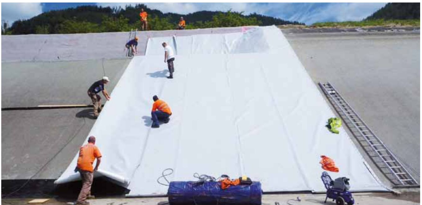
Placing of geotextile
