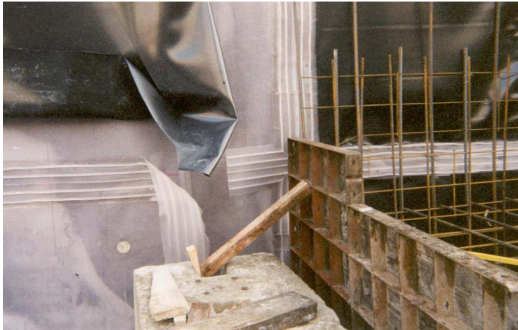
water stop installed
