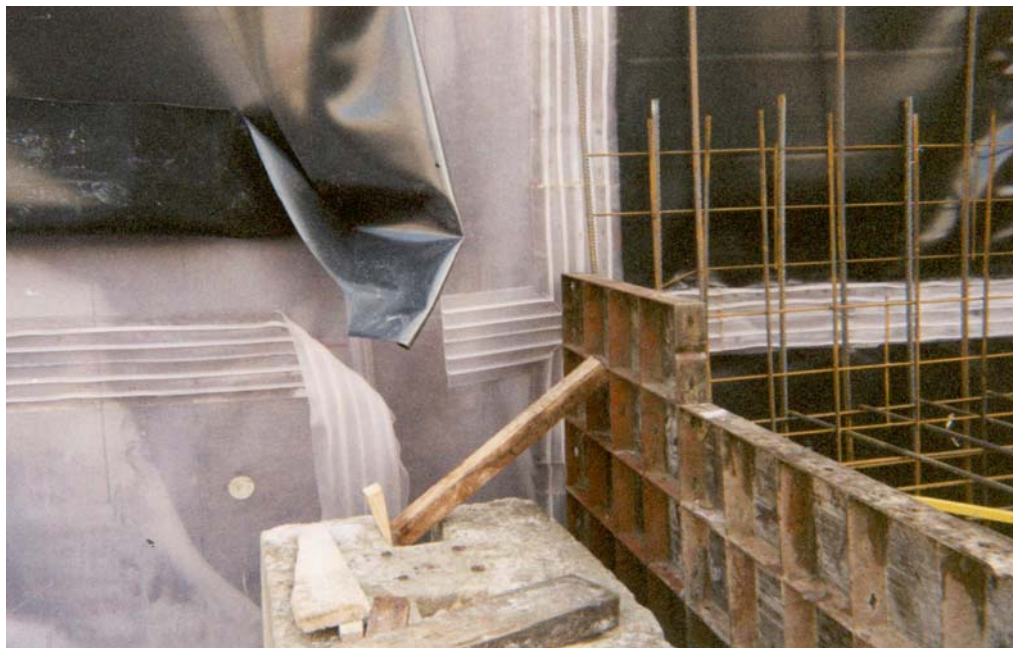
Dangers of mechanical impact to Waterproofing system
