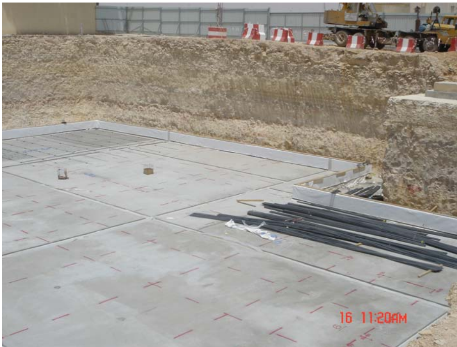
Protected Slab with exposed Water Stops
