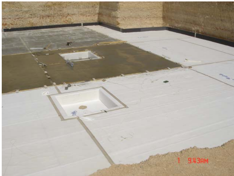
Execution of Protective Concrete
