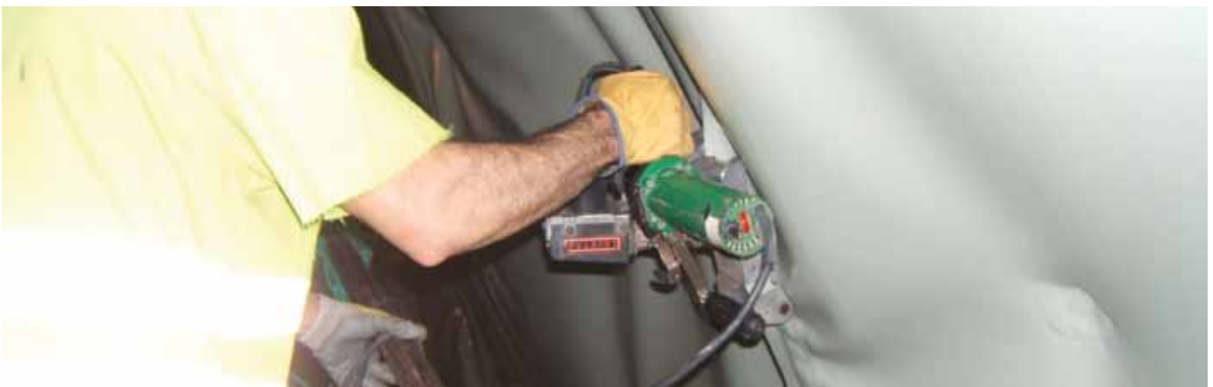
The geomembranes are welded together with automatic welding machines producing a seam with testing canal.
