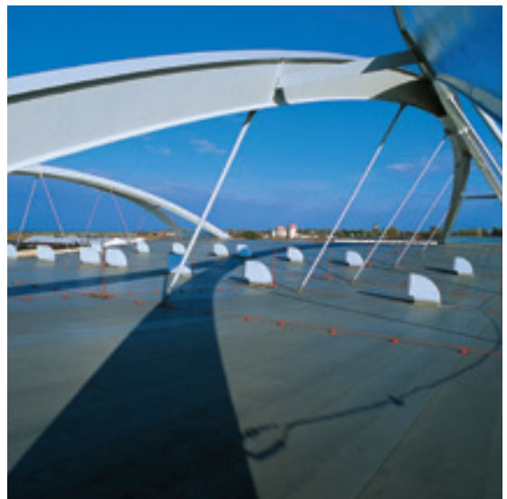
Transport station (Czech Republic)
