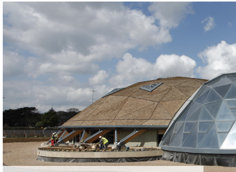
Sport and recreation centre – United Kingdom RENOLIT ALKORPLAN Solar profiles as basis for mounting cedar shingles and aluminium panels.
